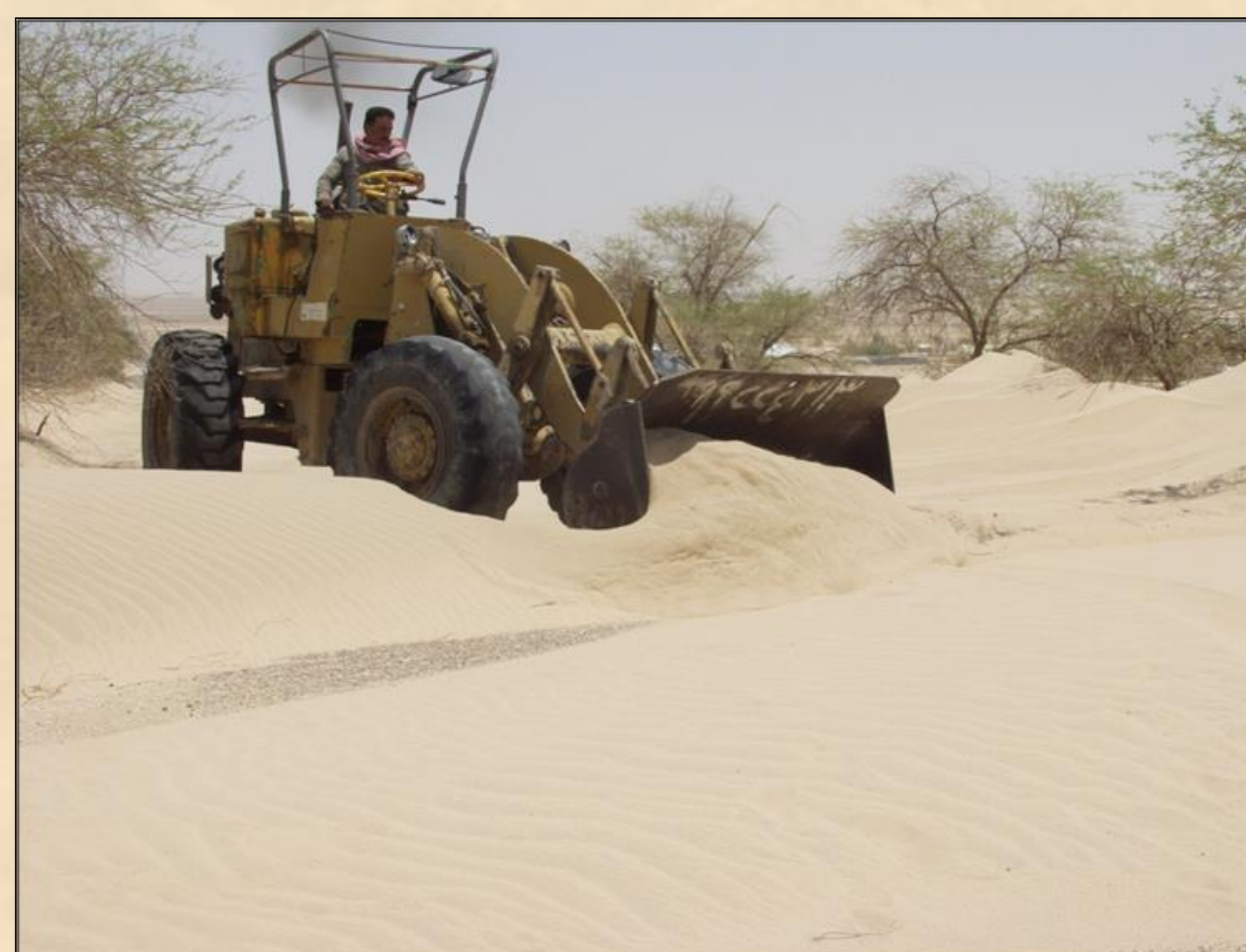
Sand deposits causing road block at Sulaibiya
